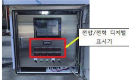
Installation of on-site monitoring panels
