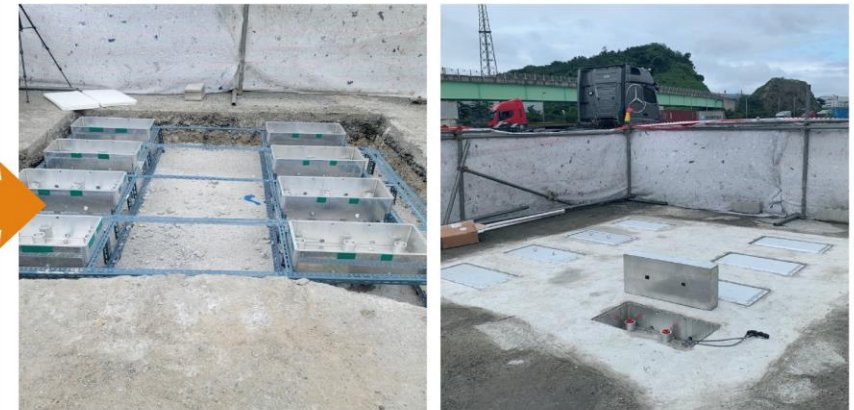
Modules after alignment and leveling work
